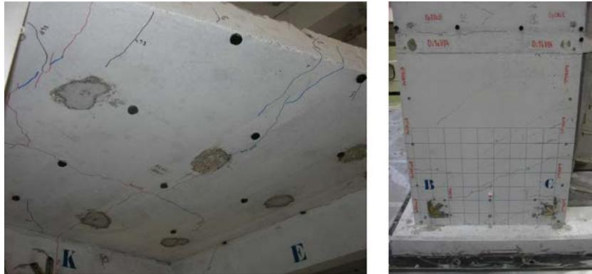
(a) Most damaged slab located at the 1<sup>st</sup> floor (b) Shear wall SW4.
