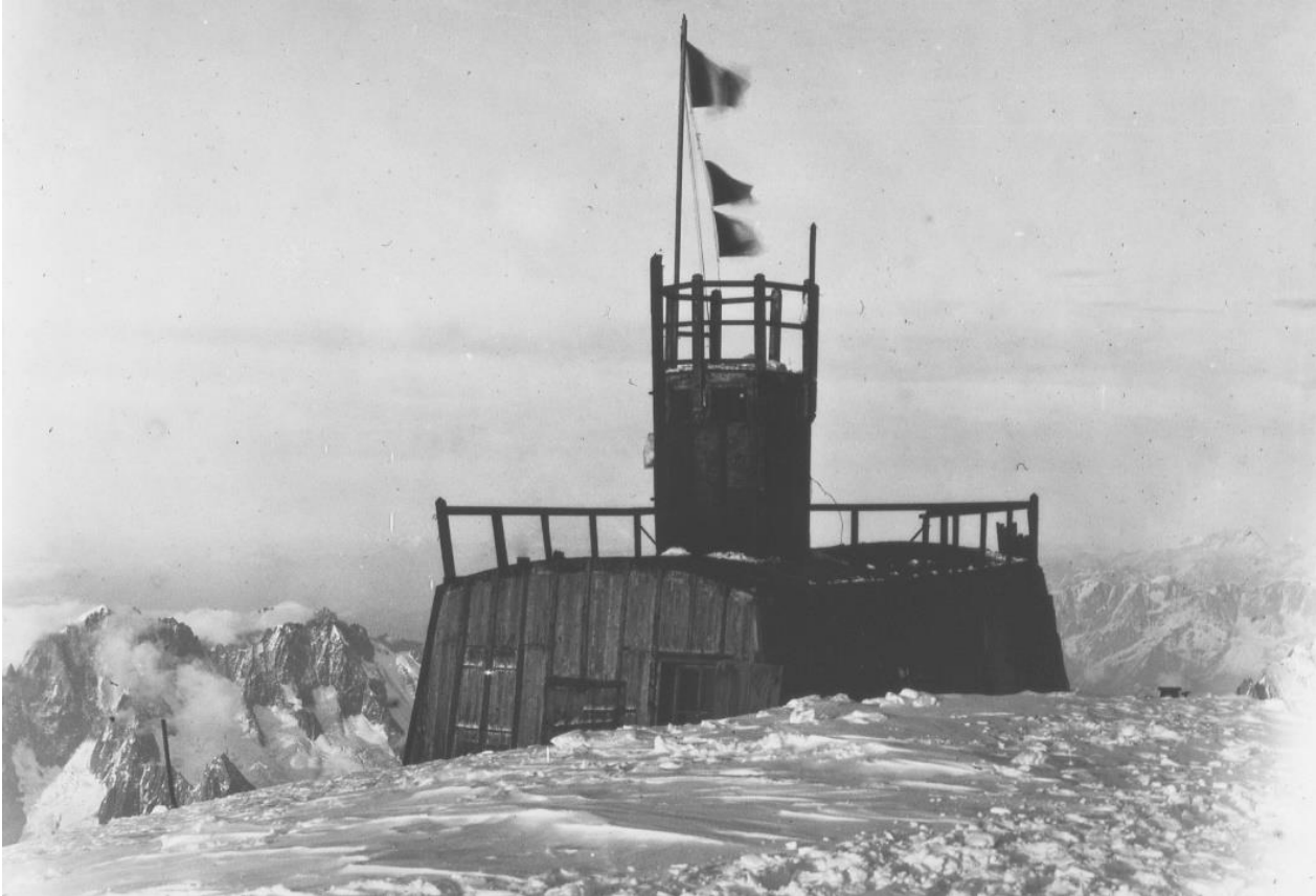
Figure 25: Mont Blanc Observatory is roughly west-east oriented on the summit crest. West and south sides appear on the photography. The refractor (not visible) is located on the northern side of the building. The observatory begins to sink slowly into the snow (courtesy Paris Observatory).
