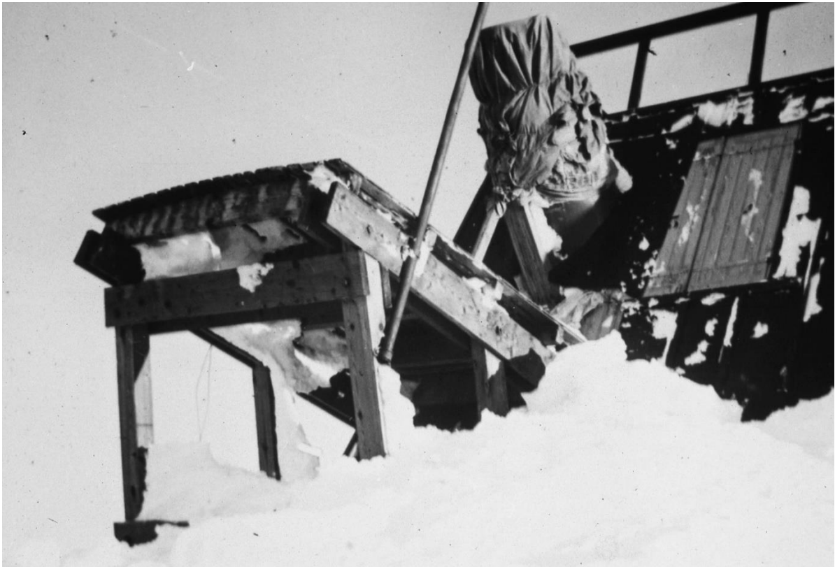
Figure 21: The 30 cm fixed-direction refractor at Mont Blanc Observatory was operational in 1896. An opening was created for the tube in the northern wall. The telescope just rotated around its axis (right ascension) to compensate for diurnal motion. The platform was used to install and remove the flat mirror of the 60 cm polar siderostat to catch the light and adjust the declination (courtesy Paris Observatory).
