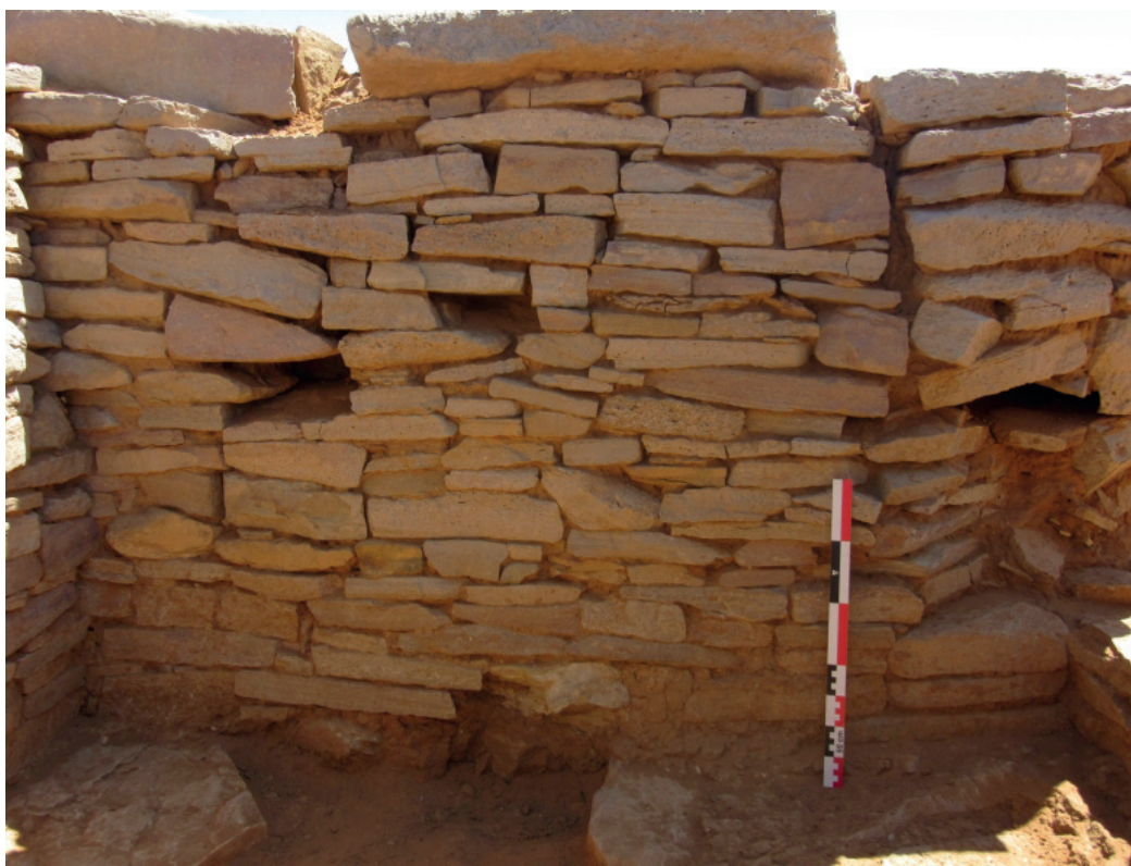
Fig. 6. Wall M3005. View to the east (DJ2016a0915b).
