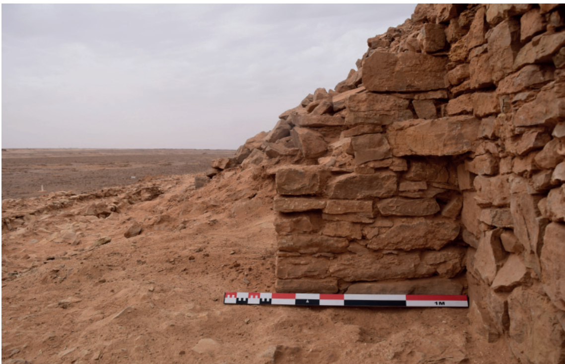
Fig. 8. View of buttress M2381 (DJ2016a0185B)
