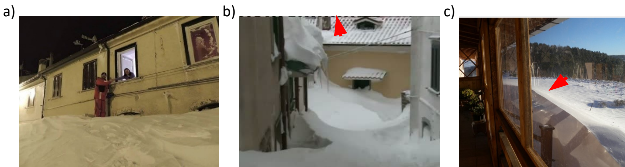
Figure 7. a) Photo of a snow accumulation due to the wind in the town of Capracotta. Photo of a snow accumulation due to wind in Capracotta (b) and Vastogirardi (c), with evidence of wind erosion on roofs and ground.
