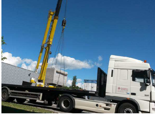
Figure 10 : Loading of the mock-up using a crane and the metal bottom support
