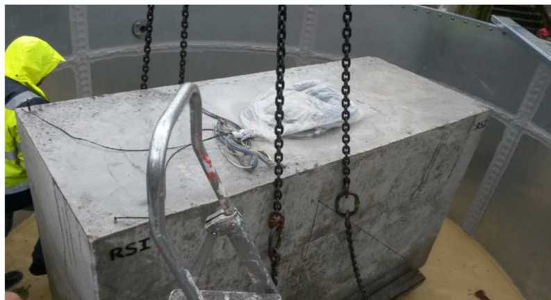
Figure 11 : Installing the DEF mock-up in its conservation pool
