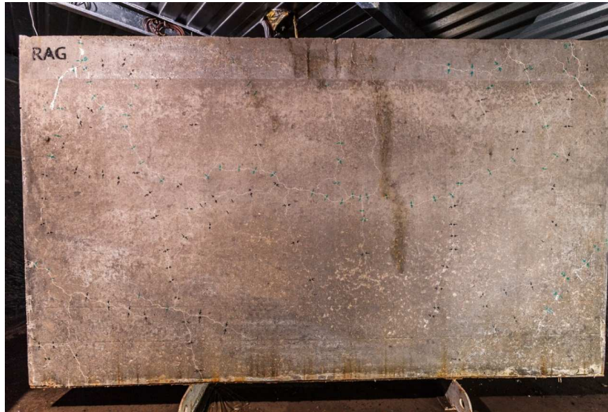
Figure 19: Photo of the ASR mock-up at t = 703 days
