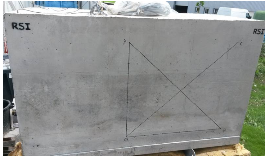
Figure 4: the axis/area used to monitor the cracking index of the DEF mock-up
