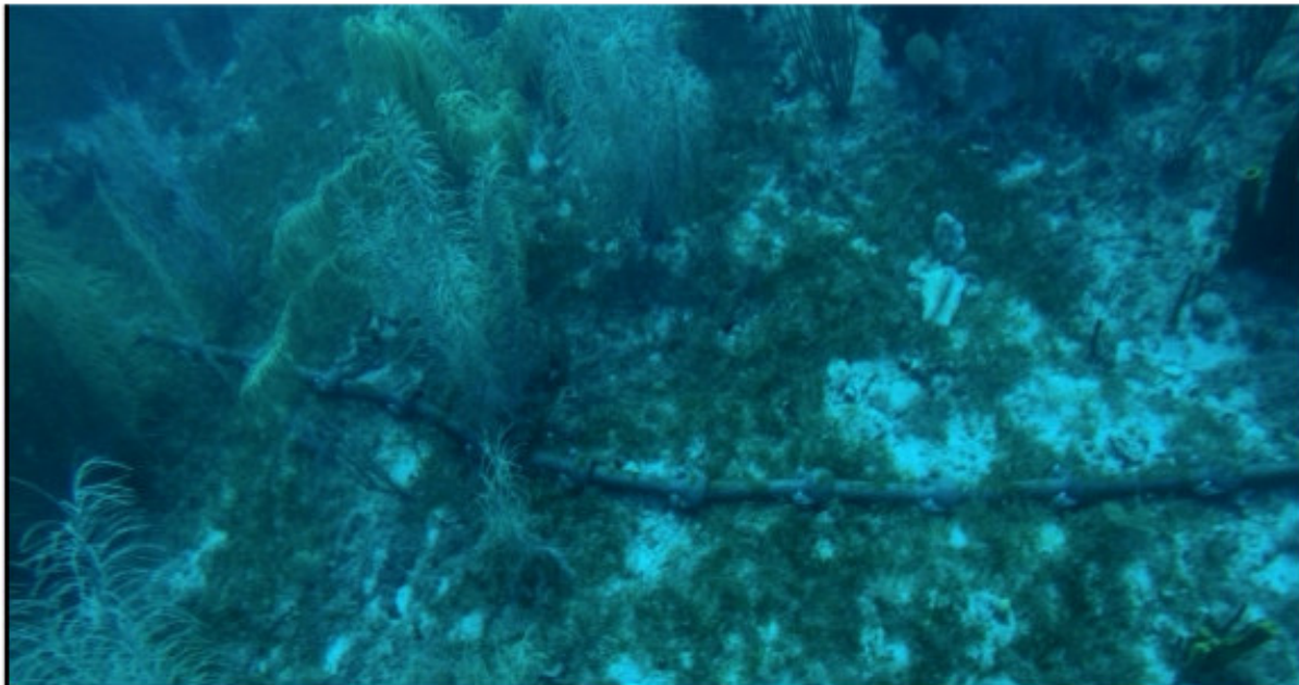
Figure 3. Landing of the cable at Anse des Mûriers harbour, Terre-de-Bas. Top: google map view of the harbour. dotted line: path of the cable protected by cast shells. Bottom: submarine view of the chain of cast shells protecting the cable.
