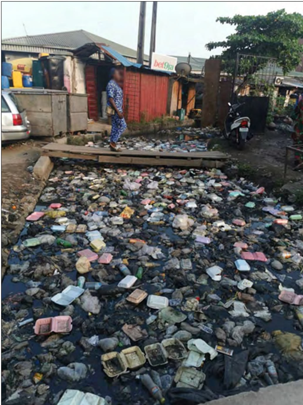
Figure 6.5 Single use plastic waste clogging open drains in Makoko, Lagos, Nigeria.
