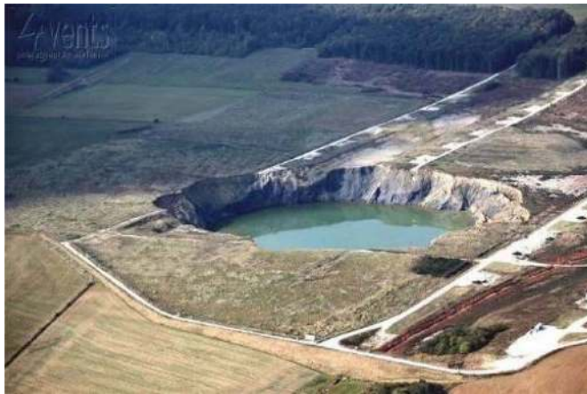
Fig. 3. The crater at Cerville-Buissoncourt six months after the collapse. (Acknowledgement: Solvay).
