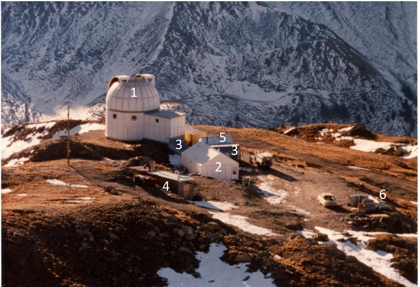
Figure 10: the station in 1977; one sees the 7-metre dome and two layer annex (1), the house (2), the double tunnel (3), the electric plant (4), the warehouse (5) and gas storage area (6) (courtesy Paris observatory)
