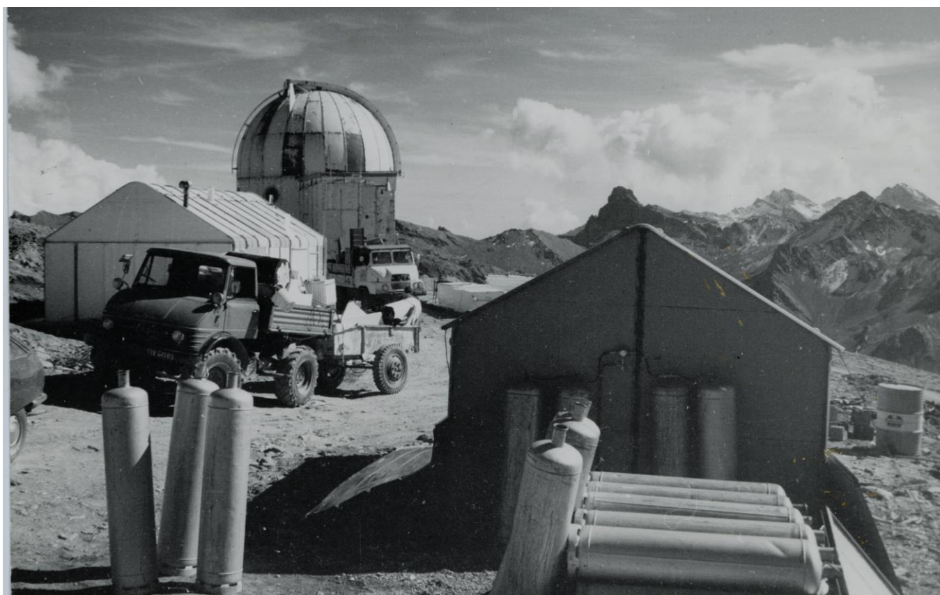
Figure 9: building the station in 1975; the heating of the house was provided by gas and electricity by fuel generators. The Mercedes Unimog 4 x 4 truck belongs to Joseph Brunet, Saint V é ran (courtesy Paris observatory)
