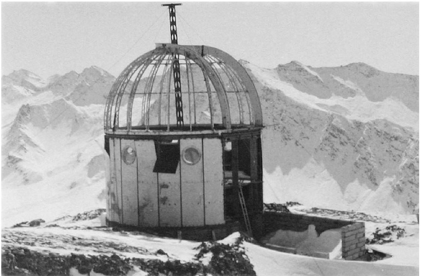
Figure 5: the reassembly of the 7-m dome during 1974 and 1975 (courtesy Paris observatory)
