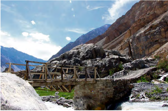
Fig. 3 (above): The "Muhabbat Trust Bridge." (Photo by the author, 2016)
