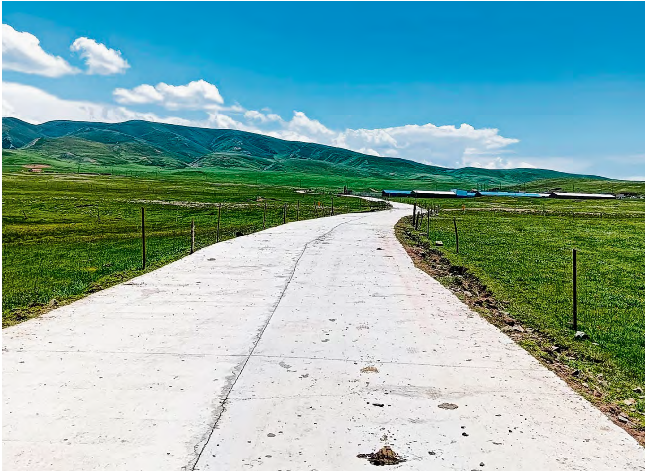
Fig. 2: Part of the new concrete road in Yangden. (Photo courtesy of Gur Gon, 2023)
