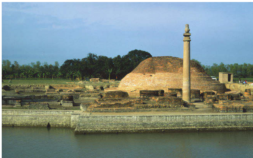
Fig. 3: The Buddhist site at Vesali with Aśokan pillar, courtesy of Harry Falk, cf. Falk 2006, 221, fig. 2.
