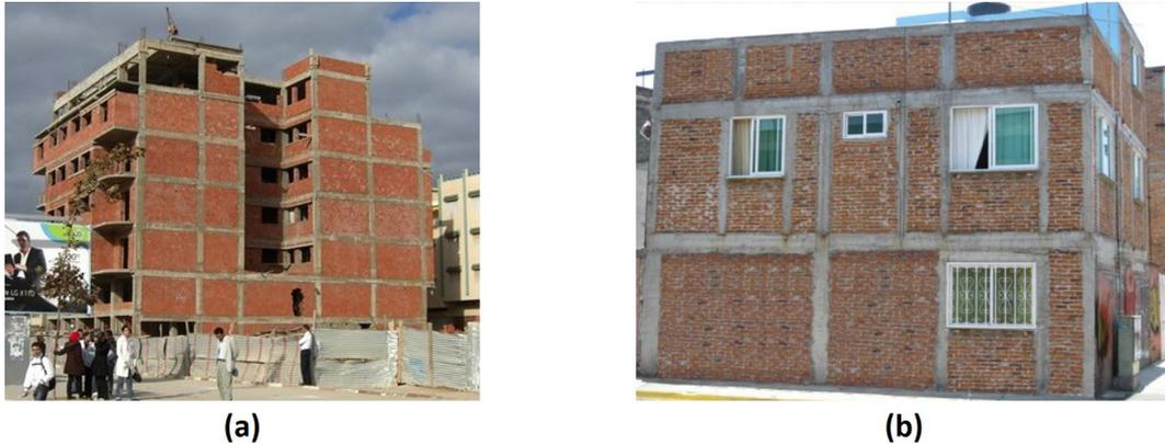
Figure 1.2: Examples of: (a) RC FIM structure (from [31]; (b) RC CM structure (from taxonomy.openquake.org)
