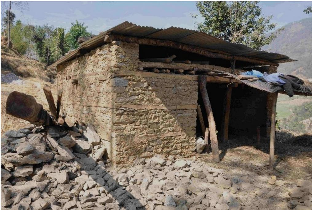
Figure 5: Masonry structure with seismic bands in Nepal
